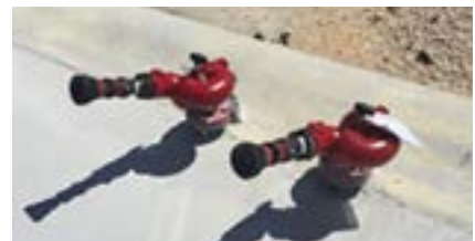
Out Rigger Monitors: Mounted at or below grade the monitors are adjustable for flow, spray pattern and direction (manual or automatic).
