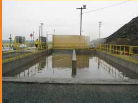
InterClean designs the wash system to handle the effluent and manage the extreme amounts of mud removed from the vehicles. Large settling pits and filtration assures we are providing high quality wash water.
